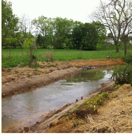
Brush mattresses sprouting on banks of Tuscarora Creek
