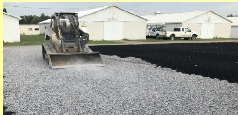
At the site now, with the work completed, the water drains to the center of the gravel lot and away from the buildings, which is what was intended
